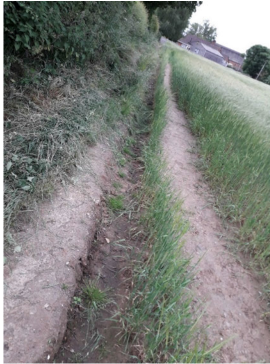
Photograph 6 – footpath narrow, rutted uneven surface
